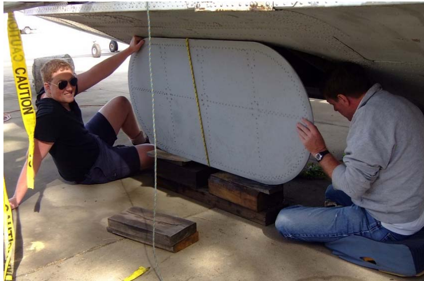
Tom Gollan (L) and friend at work on one of the water doors which is about to be removed for repairs
